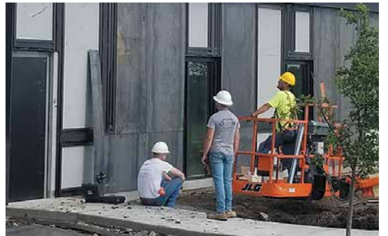
Progress is moving along at St. Luke the Evangelist Catholic School in Ankeny, where a 14,000-square-foot addition is being construction.
